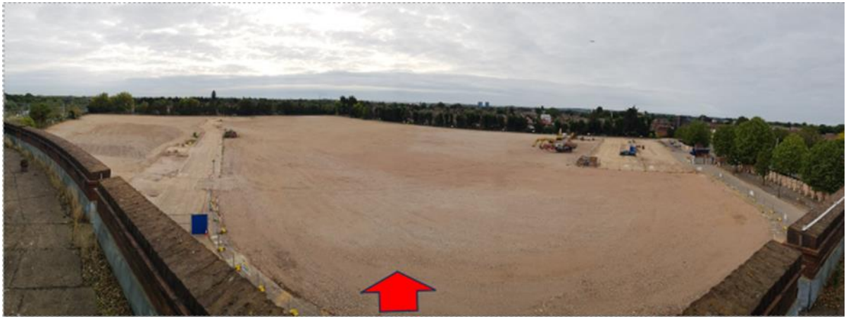
Figure 2-3 Current Site Status
