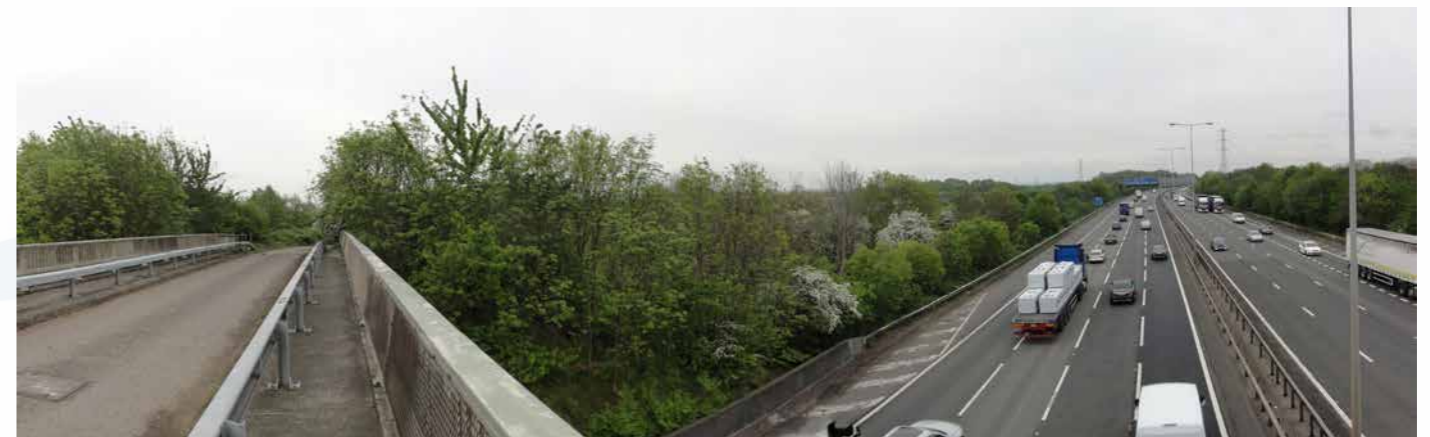
DS017 - View from Public Footpath 2 over M4 looking south-west
