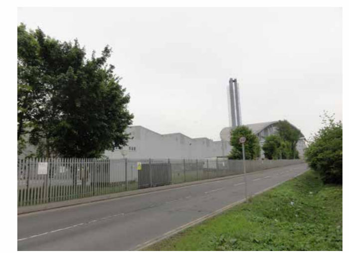
DS021 - View to existing EfW on Lakeside Rd
