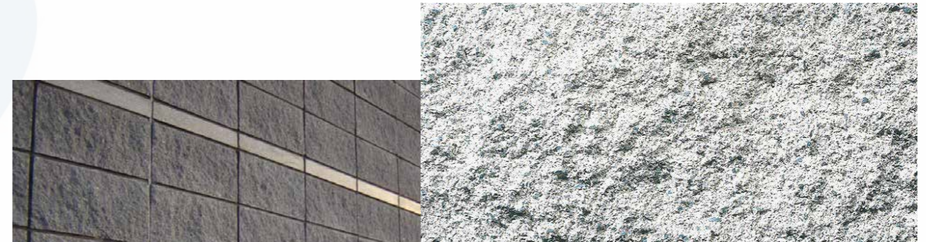
DS089 - Split face blockwork in 'Natural White'
