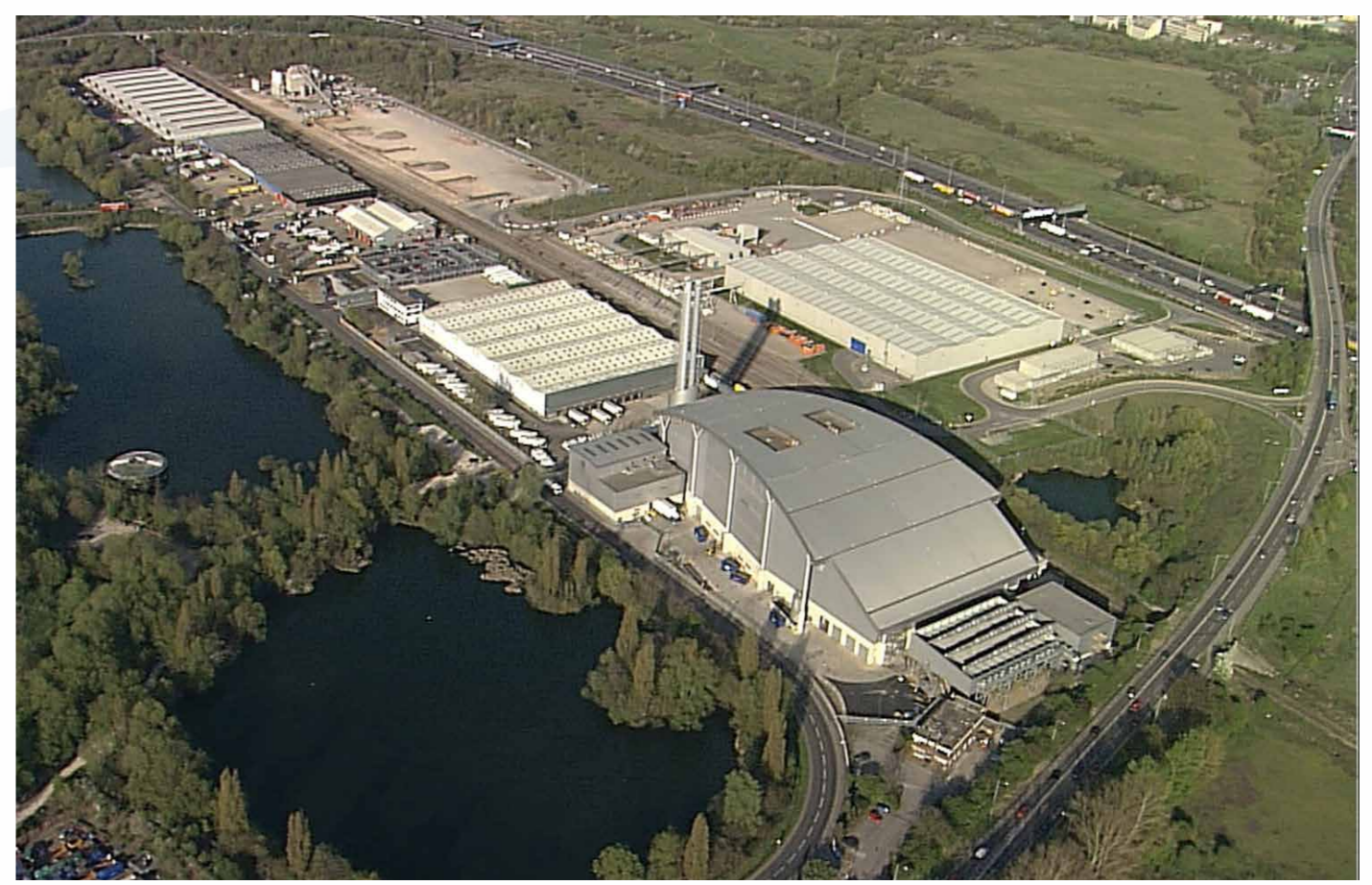
DS022 - Aerial view of existing EfW plant from south west
