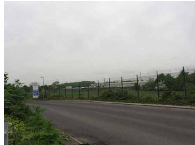
DS012 - Private road into TW sludge works
