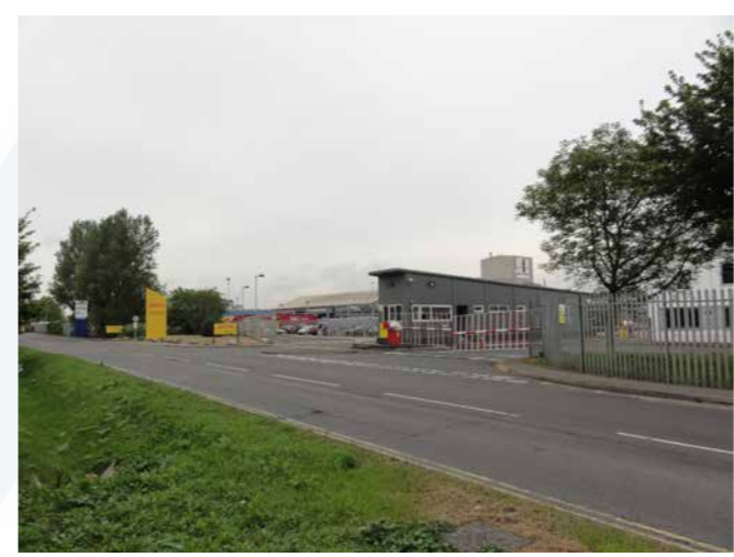
DS020 - DHL distribution centre on Lakeside Road
