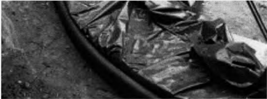
Perforated twin-wall pipes laid behind the vertical dpm
